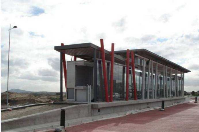
Figure 10. Trunk station on the R27 (almost complete – June 2010)
